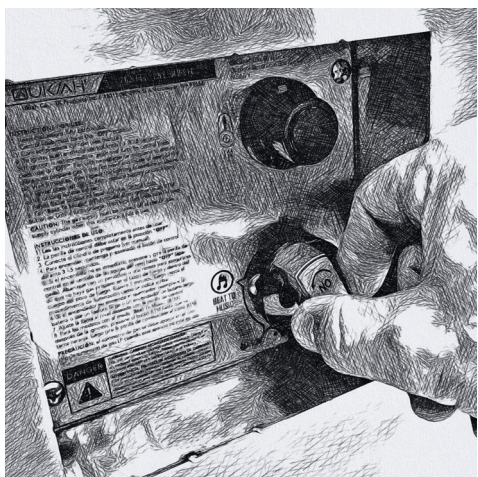
[Figure 7] - Press, hold and turn to low.
